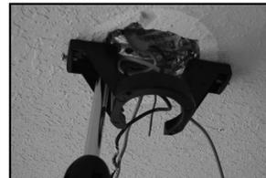
(3) Remove stopper pin and half ball from small down rod by loosening set screw on half ball. Set parts aside for reinstallation in step (7).
